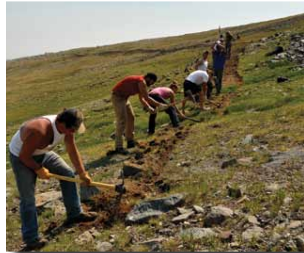
Ben Gleason of Billings makes the first cut as other members of the volunteer trail crew follow, widening the new trail.
