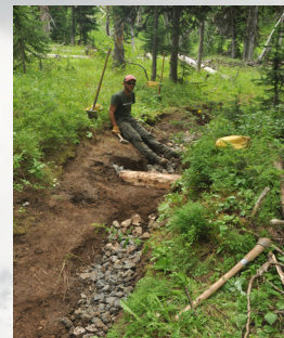
Filling in a deeply rutted Lake Abundance Tr.
