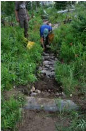
Karen Holcomb and Linus Metzler fill in the entrenched trail with rock and soil
